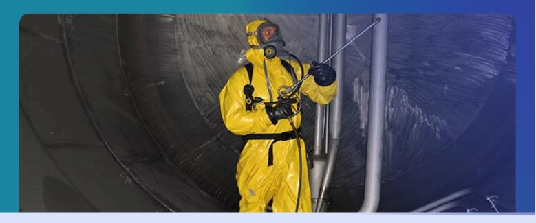
We provide fast, efficient and safe disludging and cleaning services for FPSO using automated cleaning system with High Pressure Jetting and Vacuum Transfer System capable of water jetting and cleaning of the interior surfaces, and evacuating mud from a depth of over 50meters in FPSO.
